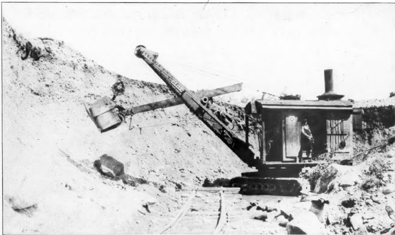
View of Steam Shovel, showing also Character of Gravel Bank
